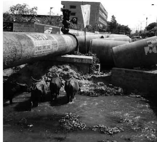
Fig. 1 Photograph shows the sewage water pipeline is one of the potential hazards causing H. pylori transmission in India. The pipeline is leaking near the gutter and the buffalos are grazing in it. This is a common picture in most of the cities in India presenting the view of water contamination and transmission of water-borne diseases.
