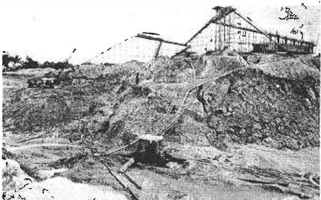
Fig. 2 View of pump shed, 'palongs' (sedimentation units) and hoppers.
