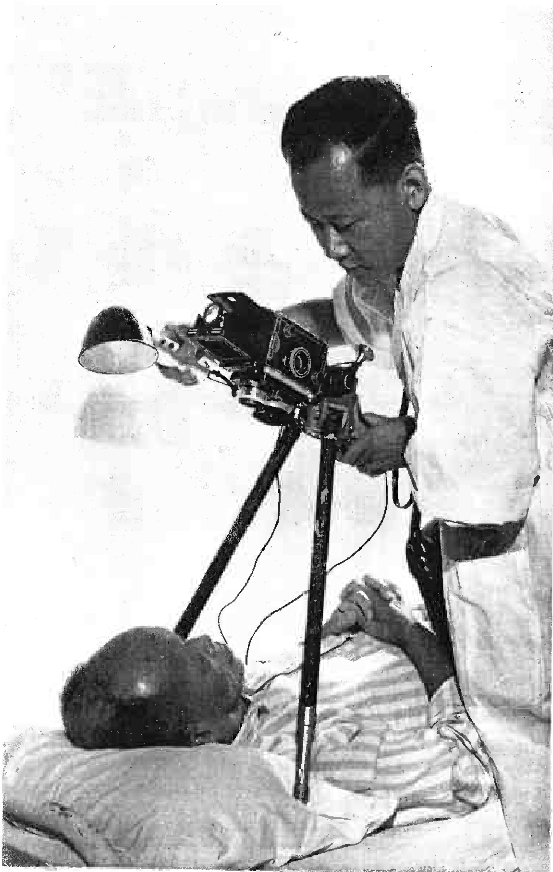
Figure 9. Photo shows the use of a "Bipod" for close-up work in the ward. This "Bipod" is specially made for bed ridden cases where the setting up of a tripod is a problem.
